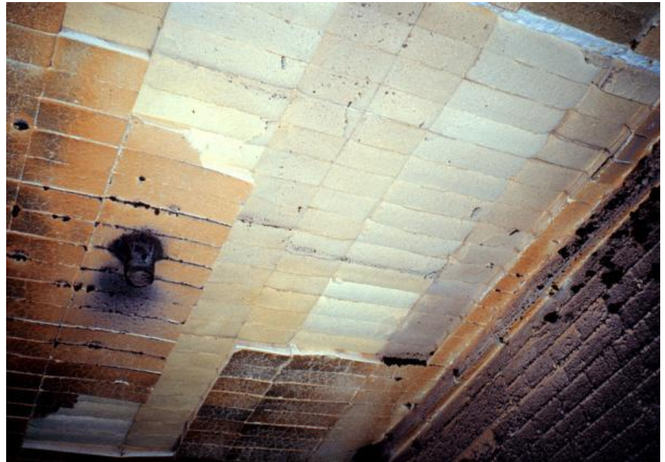
Showing Surface Glazing and Sheet Spalling
