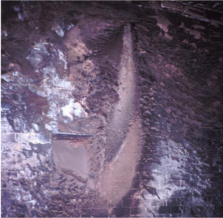
Sidewall of Sawdust Fired Tunnel Kiln After Seven Years of Service
